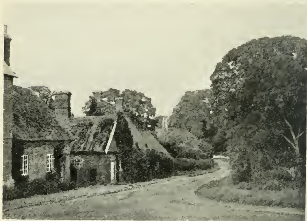
Typical Leicestershire Cottages at Scruptoft
